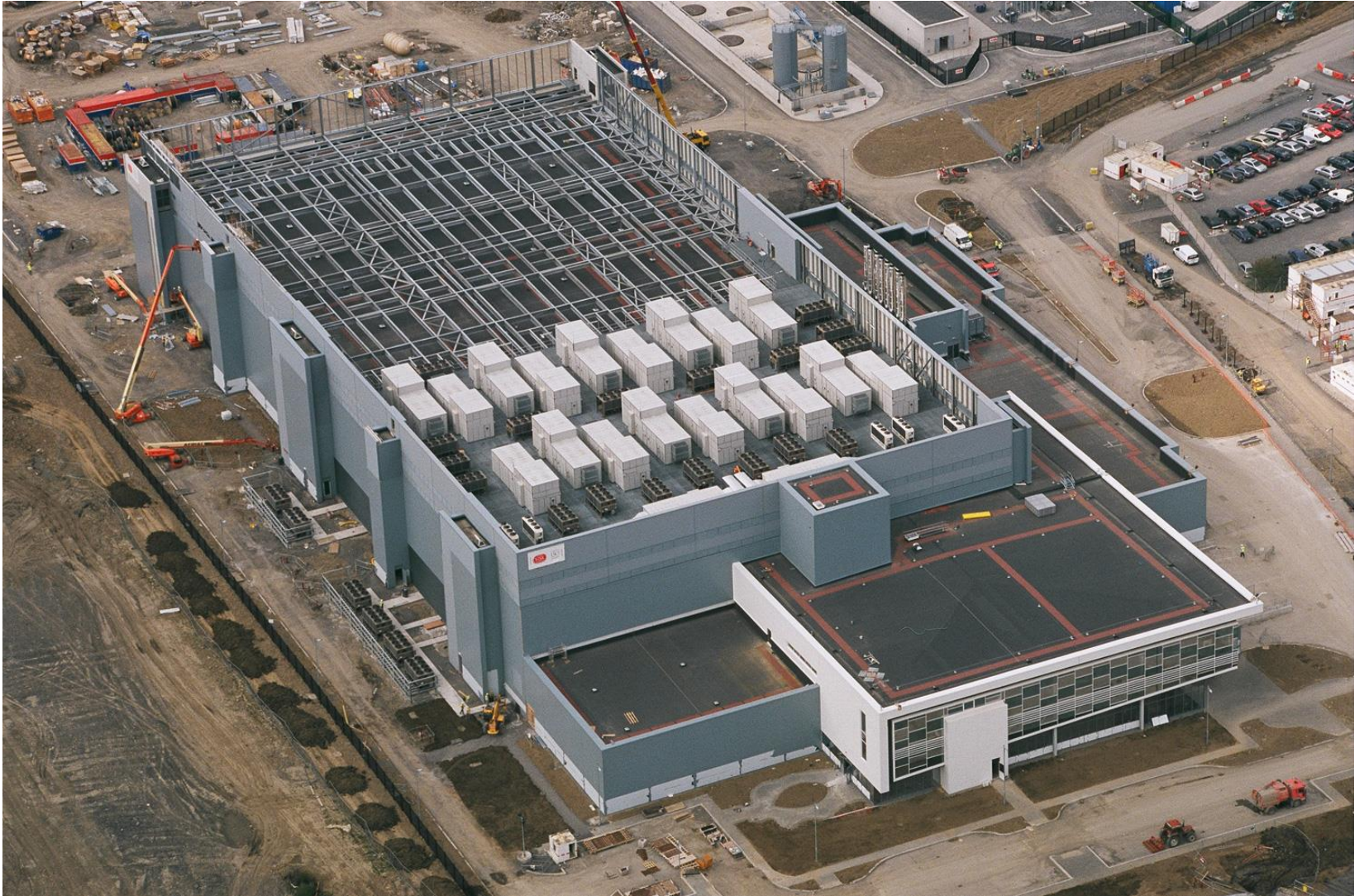
Microsoft's Data Center in Ireland
