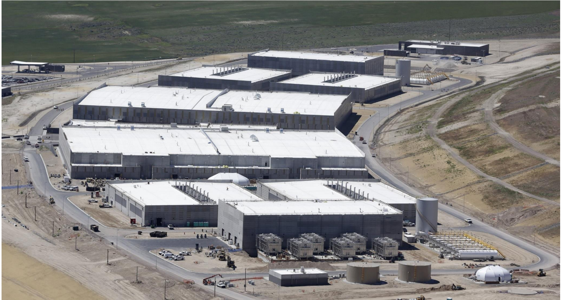
NSA's Data Center in Utah
