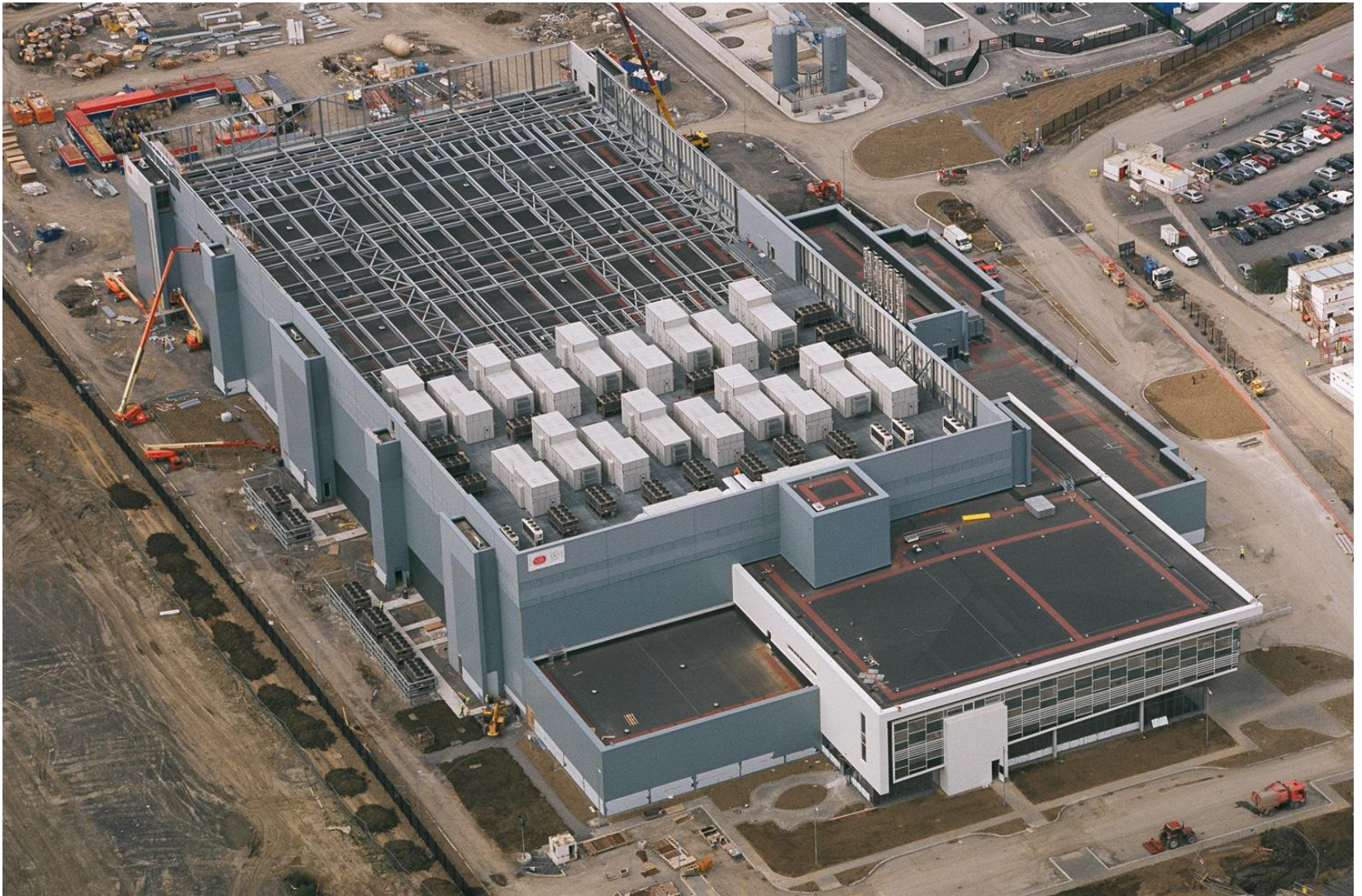
Microsoft's Data Center in Ireland
