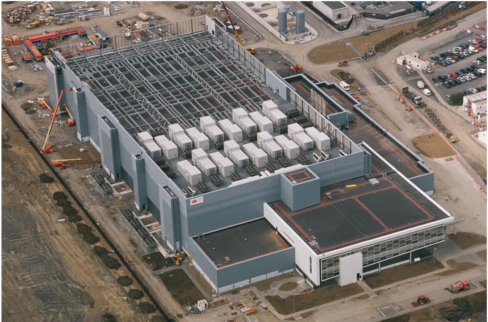
2017-01-17 Microsoft's Data Center in Ireland
