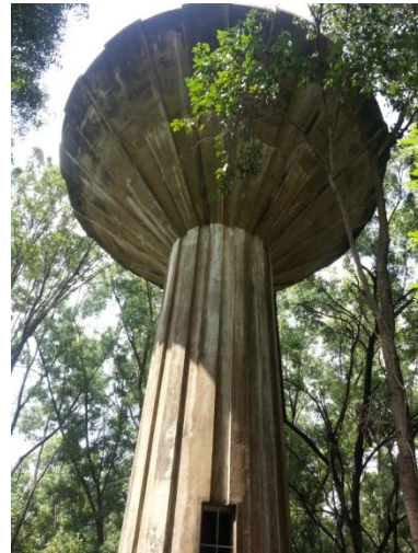
Behind old C- Mess
